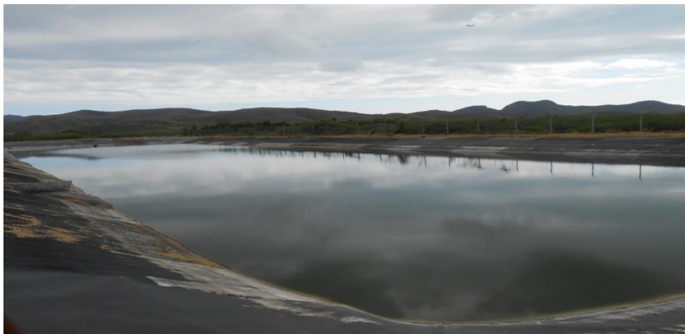
Fig. 1.14 Leachate pond at landfill
